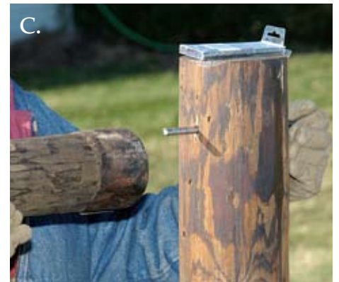
Inserting the Brace Pin and the wood brace post.
