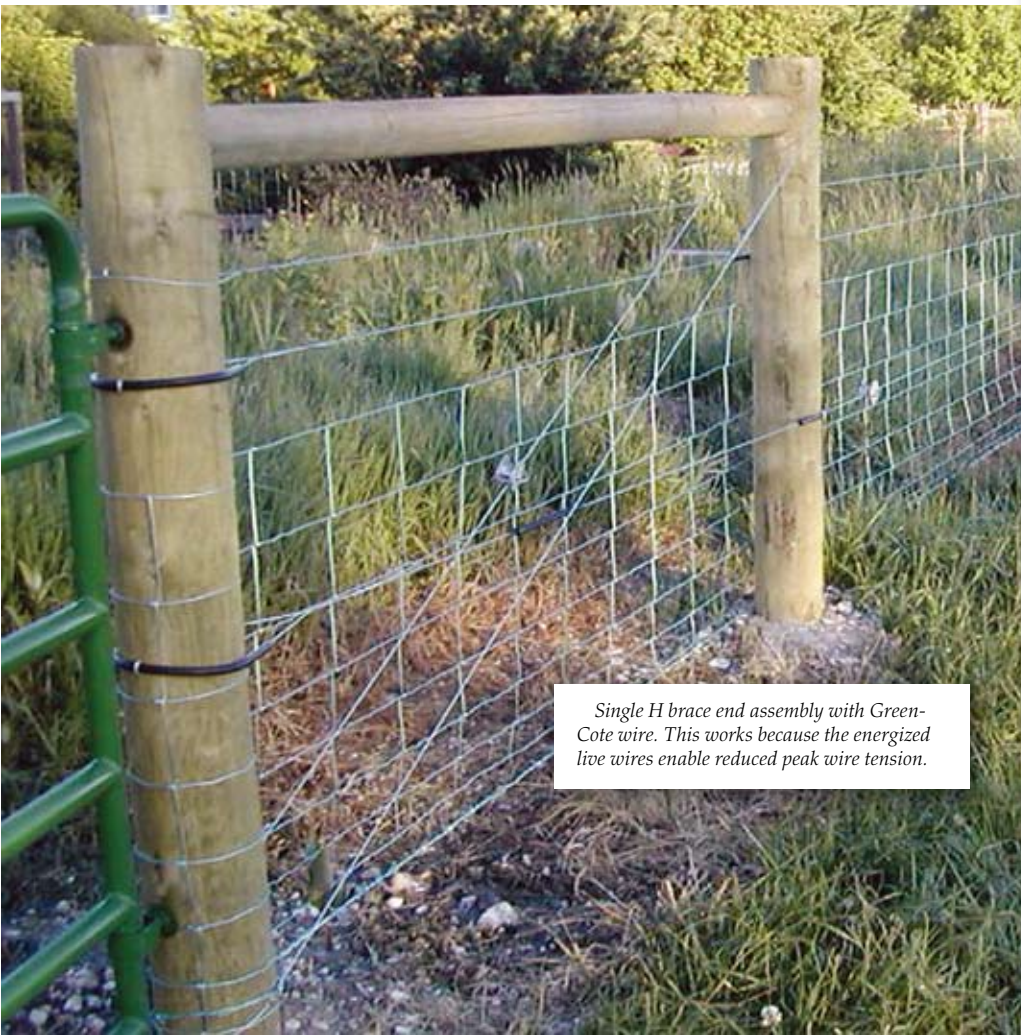
(above) Single H braces on the corner of a woven wire fence at Premier.
