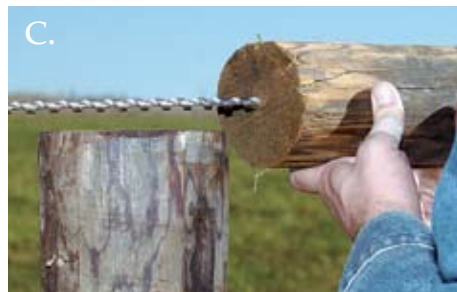
Drilling a hole in the center of the wood brace post.
