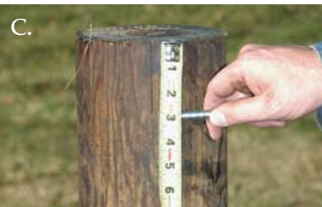
Measuring 3 in. down for installation of Brace Pins.
