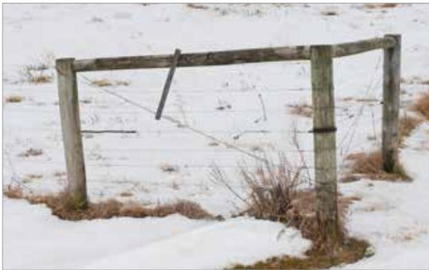
*Cross brace is too short and set too high—allowing end post to be pulled out of the ground by the tension of the wire fence*
