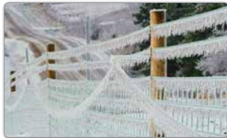
Heavy ice/snow can weigh down electroplastic conductors. When this occurs, turn off the energizer and break ice off the conductor. Sagging stretches and wears the plastic and metal filaments.
