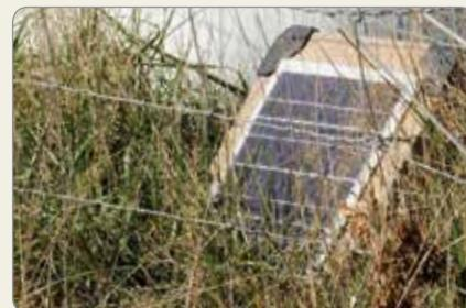
**6. Allowing posts, grass (above) or trees to shade it for a portion of the day.** If a solar panel is not **fully exposed to the sunlight all day, it won't develop enough voltage to recharge the battery.**
