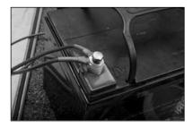
3. Unscrew the bolt of the red "+" battery terminal. Make sure to keep the lock washer and regular washer on the bolt. Remove red tape from red "+" wires. Bolt "+" wires into the terminal. Tighten bolt until all components are firmly touching each other.
