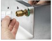
3. Pipe tape may be required between a/b connection.
