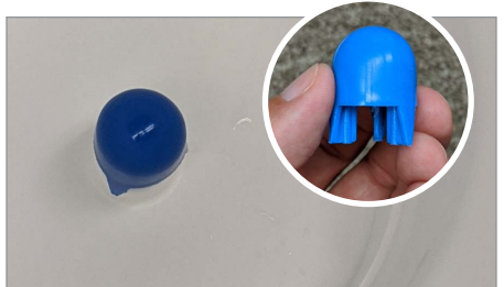
7. Valve Cover installed inside the water tank.
